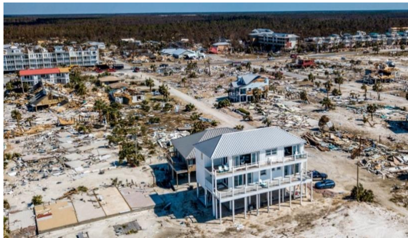
Figure 1-2. Buildings still standing in Mexico Beach after Hurricane Michael, 2018, picture courtesy of the New York Times 2 (Mazzei, 2018)
