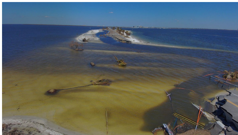
Figure 7. Hurricane Ian Damage to Sanibel Causeway (FDOT, 2022)
