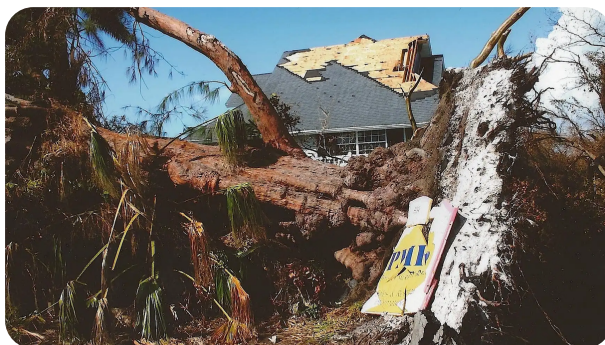
Figure 4. Hurricane Damage on Captiva Island
