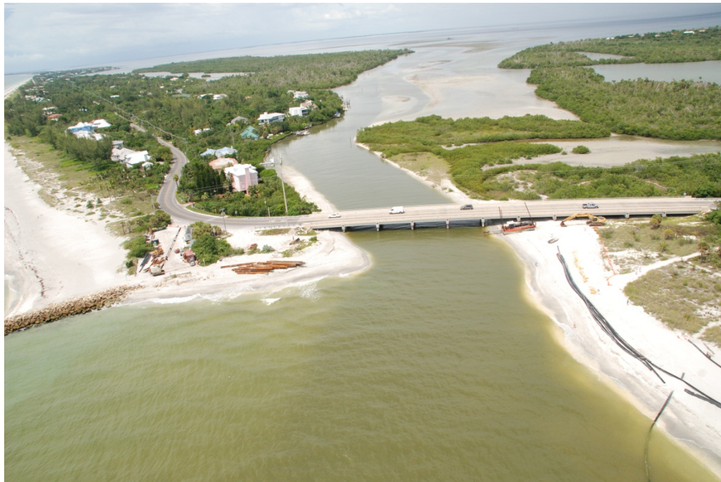
Figure 2. Aerial photograph of Blind Pass after opening (August 2009)
