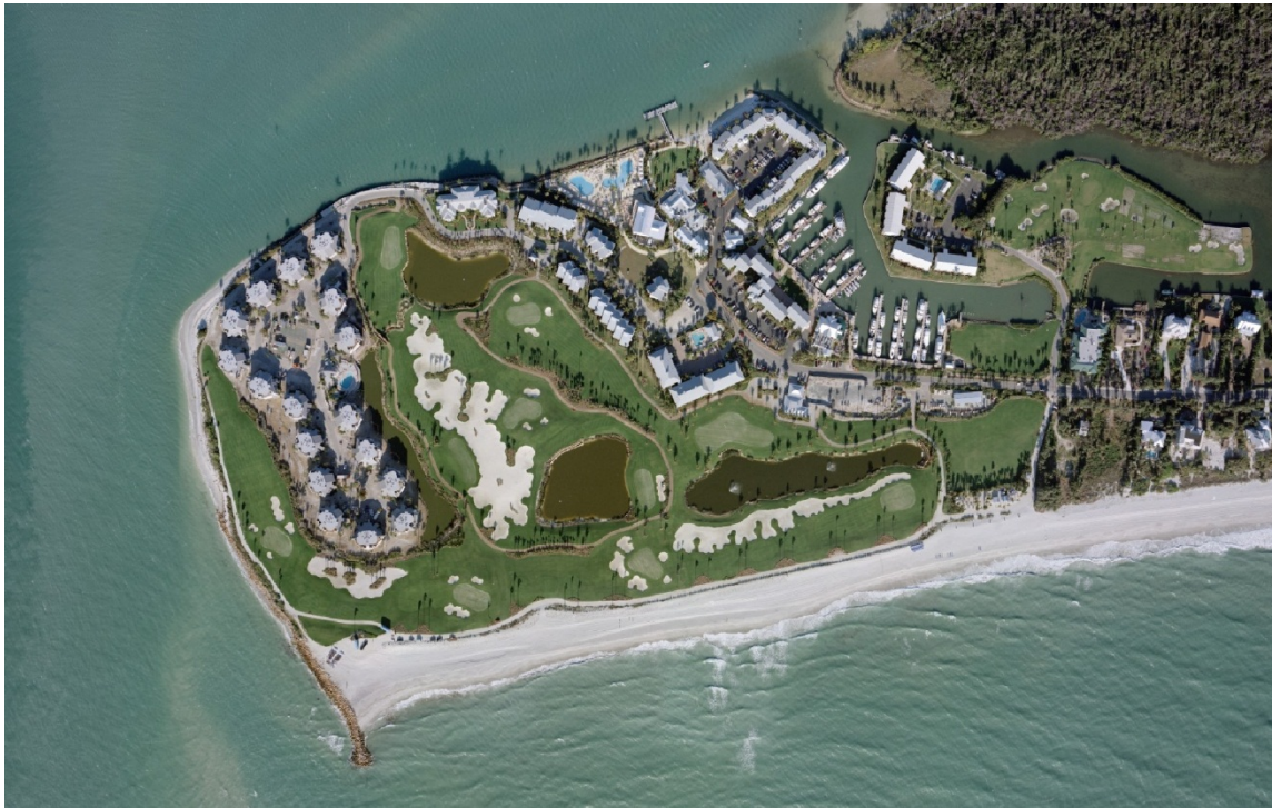
Figure 3. Captiva Island Adjacent to Redfish Pass after the 2006 rehabilitation and extension of the terminal groin
